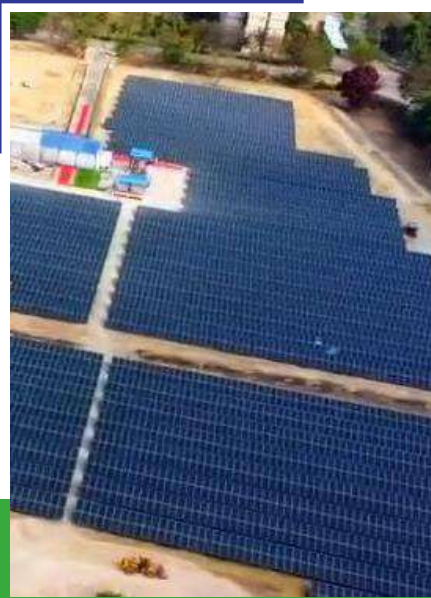
6.5MWp Ground Mounted Project at Raigarh, Chhattisgarh
