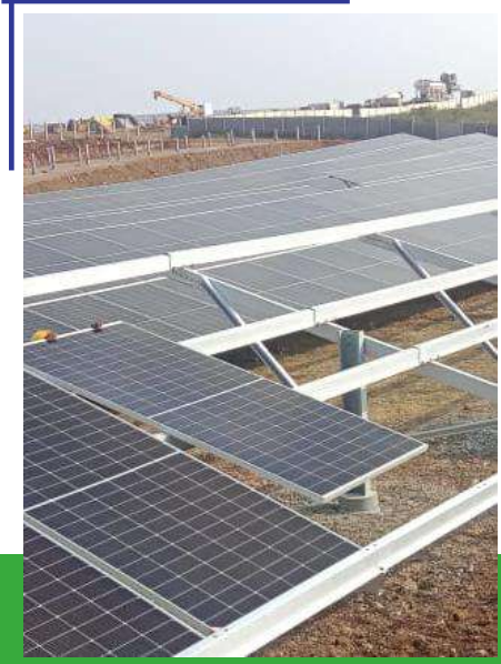
150MWp Ground Mounted project at Ratlam, Madhya Pradesh
