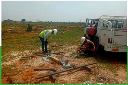
295.68MWp ground mounted project at Kurnool, Andhra Pradesh
