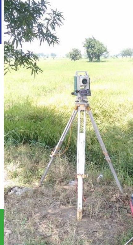
6.5MWp groundmount Project at Raigarh, Chattisgarh
