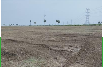
154MWp ground mounted project at Thoothukudi, Tamil Nadu
